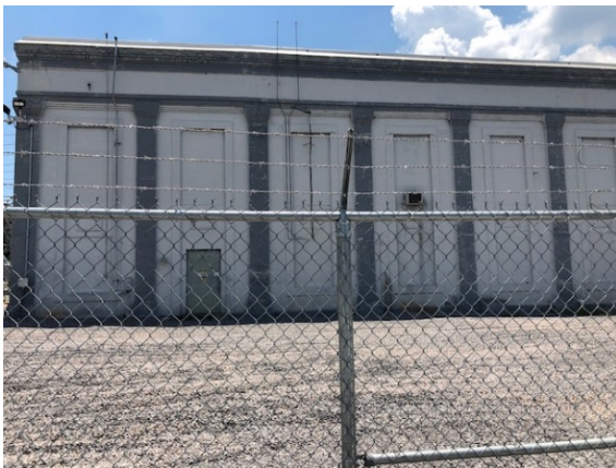
Type 3: Metal with Overlapping Panels
